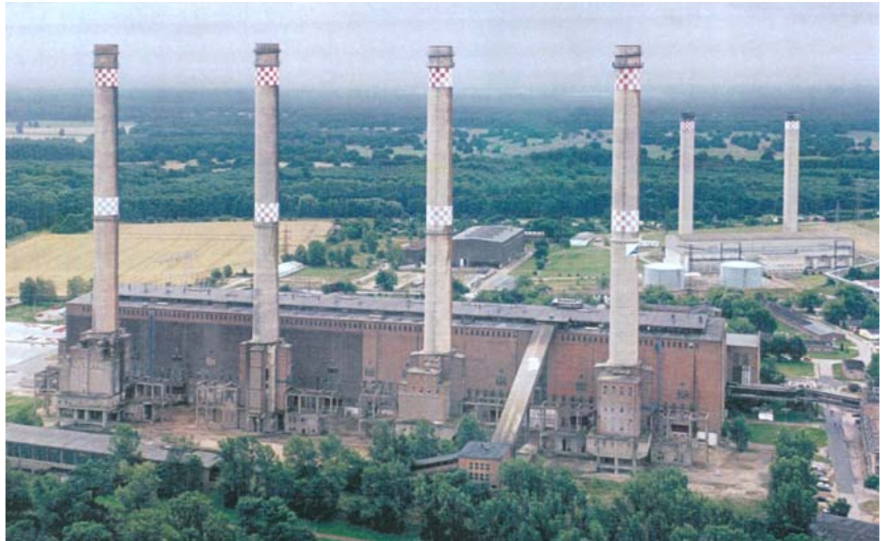
Power station Vockerode before detonation
